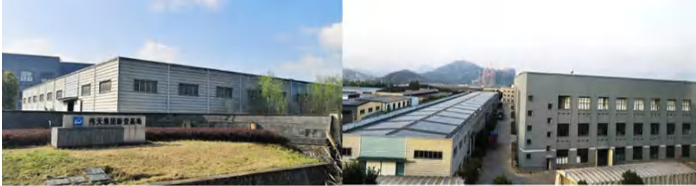
Weitian Factory Buildings - Around 90000 SQM
